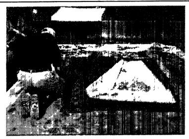
N Applying grout to the inner SDRI ring installation
