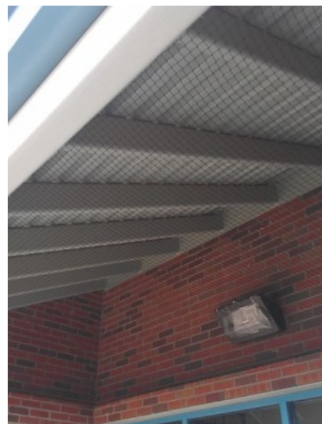
Meshed netting was used on this military building to keep Western Kingbirds from repeat nesting on the light fixture.
