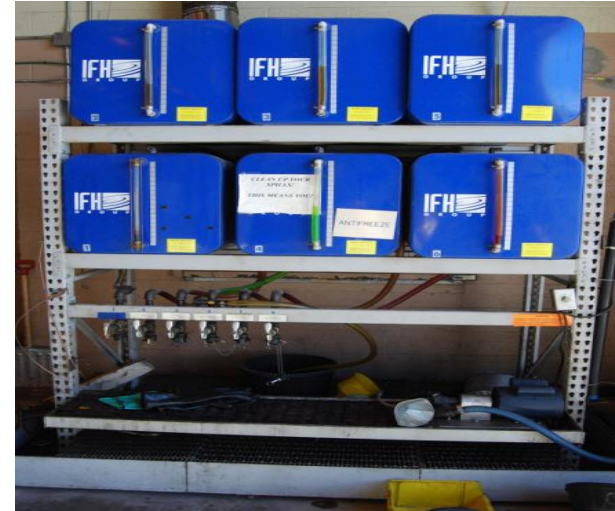
POL distribution with containment
