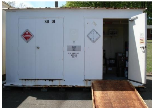
Conex with built-in containment
