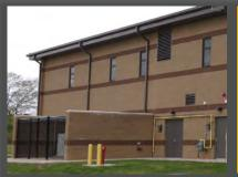
Left: Building 71371 is constructed with brick and incorporates a low pitch roof. The mechanical system is located to the side of the facility and is screened and fenced for safety and aesthetics. Below: Appropriately sited landscaping outside the 5th Special Force Group (SFG) Barracks ensures limited maintenance and provides a healthy environment for the tree to mature and arow.
