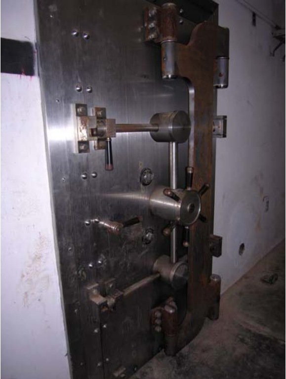
Figure 9. Door securing storage cell (Gatewood and Doerrfeld 2008).
