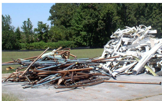
C&D Debris Segregated for Recycling
