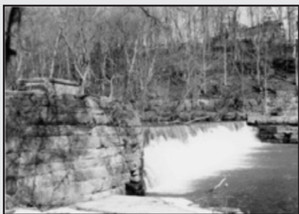
The mill dam at the Ringgold Mill, located on Little West Fork Creek just outside of Fort Campbell. The dam directed water from the creek into the mill race. The race funneled water to the water wheel or turbine that powered the mill.
