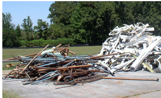
C&D Debris Segregated for Recycling
