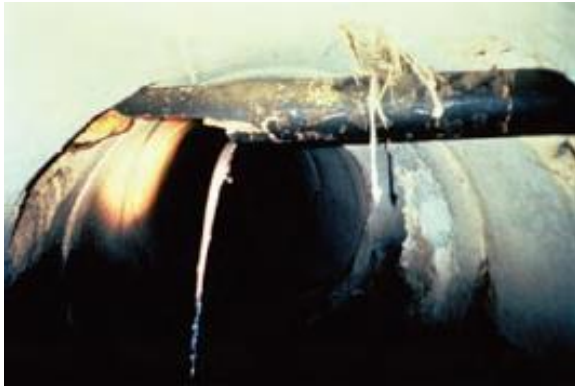
Sewer Pipe Leaking into a Storm Pipe
