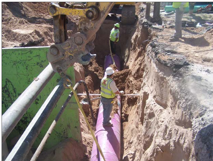
Figure 2-3. Installation of Purple Pipe in City of El Paso
