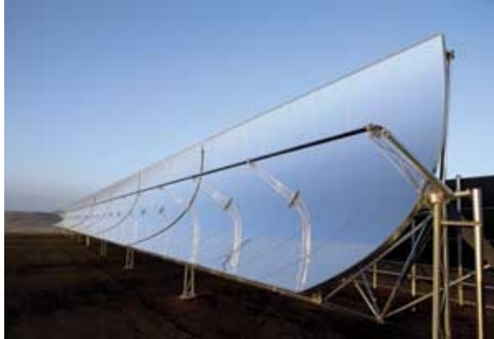
Figure 2-7. Concentrating Solar Power Parabolic Trough Technology
