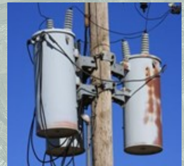
Typical PCB-containing Transformer
