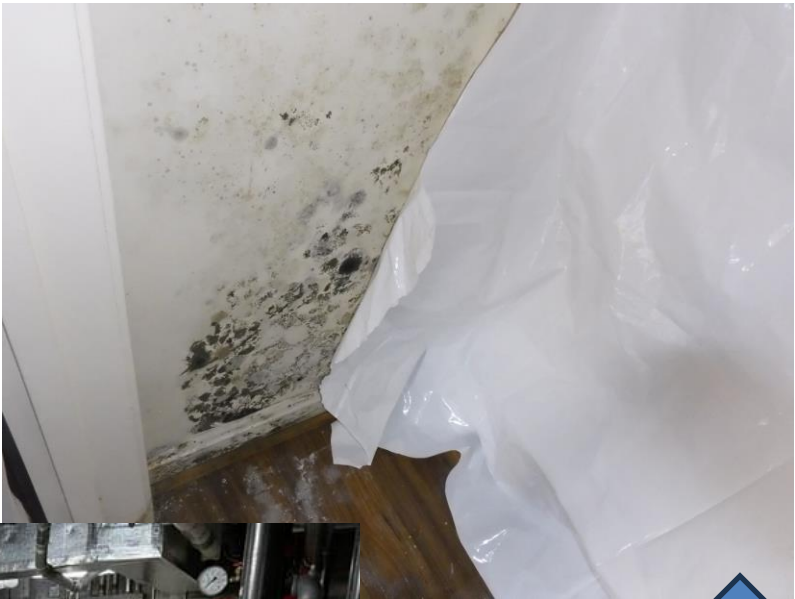
Pipe leak on other side of wall
