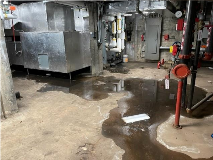
Overflowing drip pan
