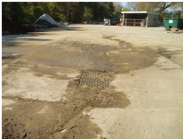
Unprotected storm drain inlet
