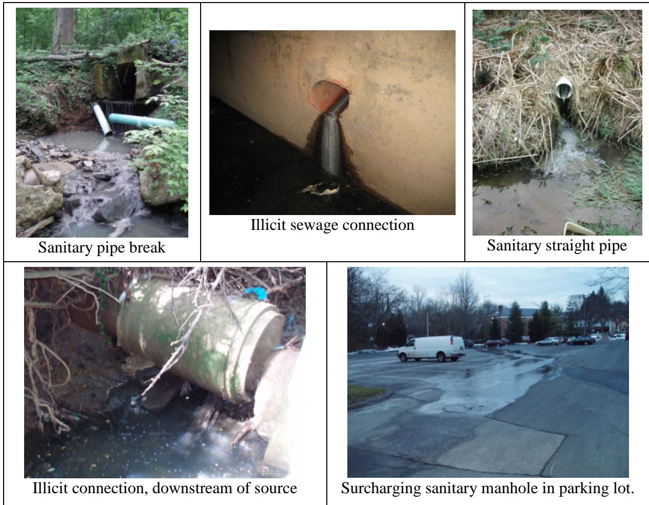
Figure 8-5 Sanitary Sewage Discharge Sources
