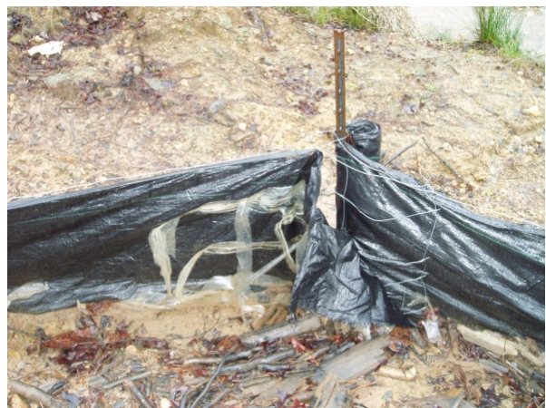
Failing silt fence
