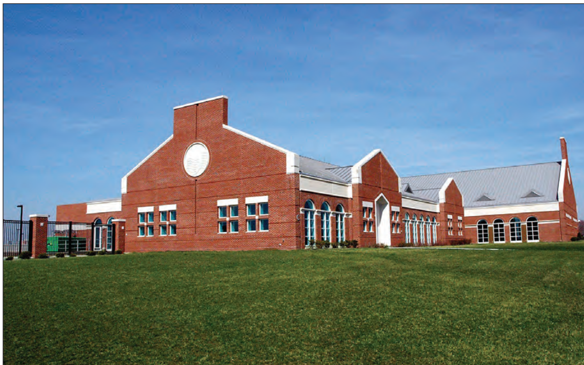
Fairfax Water's Frederick P. Griffith Jr. Water Treatment Plant
