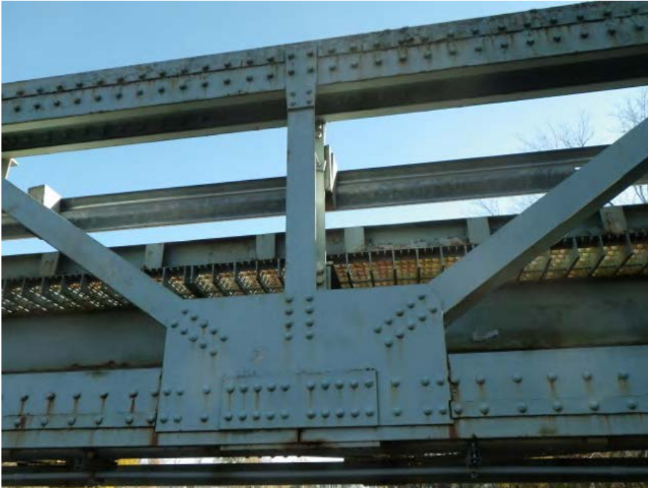
Typical Truss Vertical/Diagonal/Gusset Plate Connections
