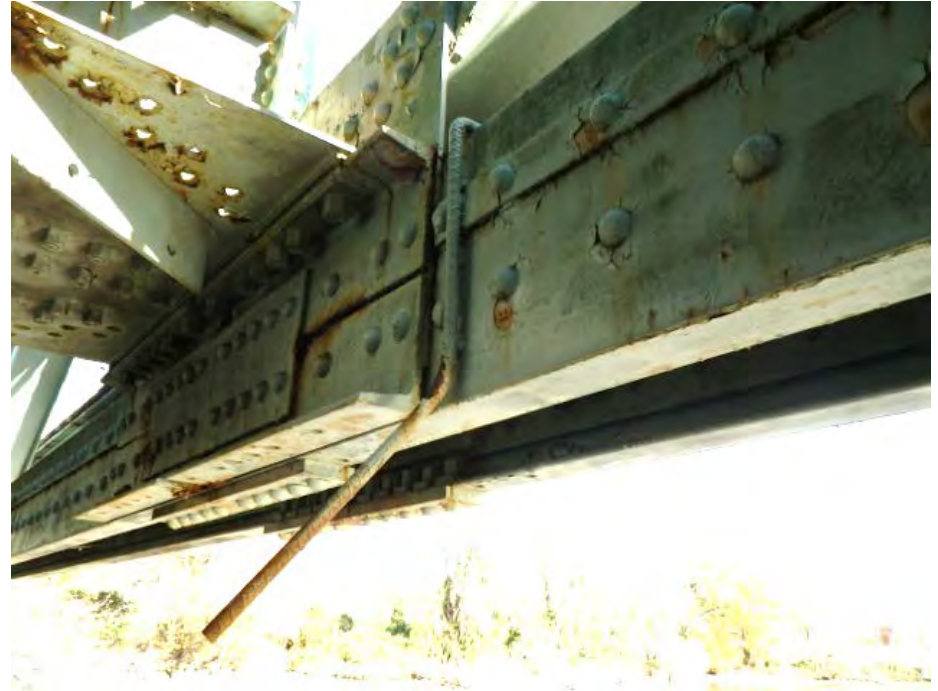
Random sections of rebar welded to lower chord (Fatigue Category C)
