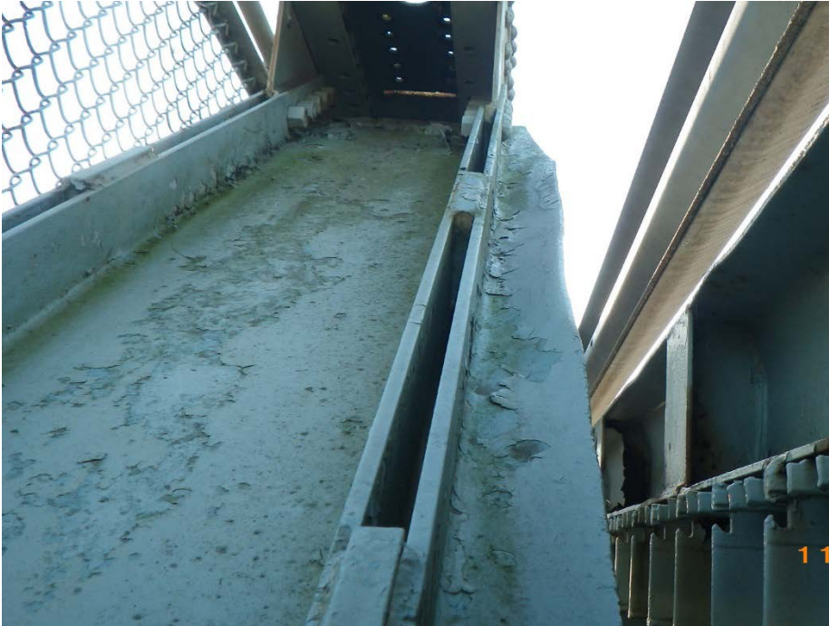
Welded Spacers Between Built-Up Diagonal Members (Fatigue Category D)
