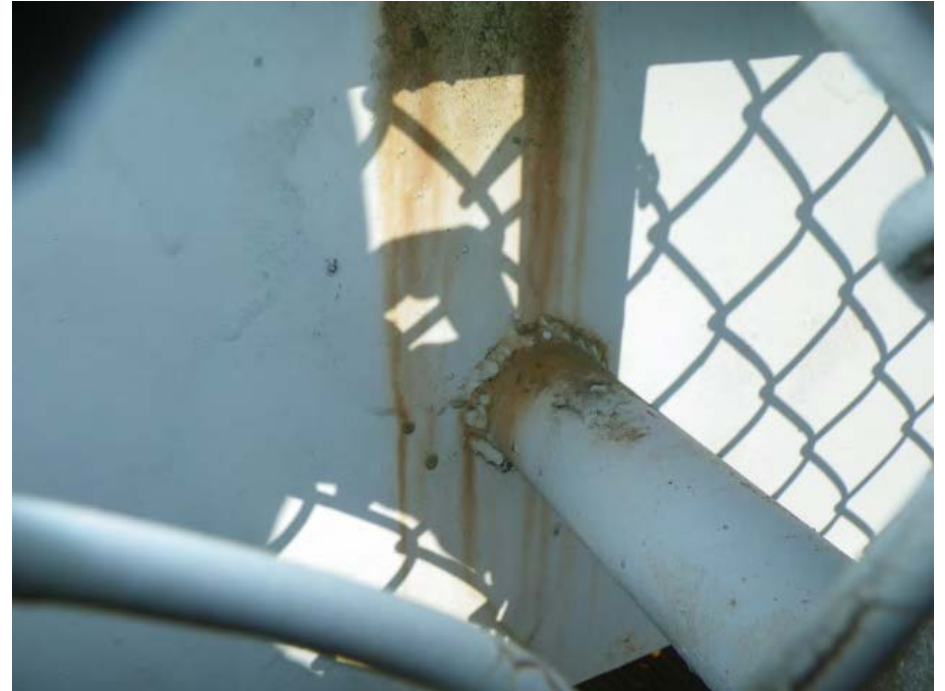
West Sidewalk Handrail Welds to Truss Diagonals (Fatigue Category C)
