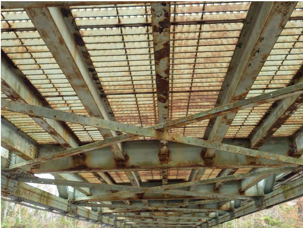
Figure 12. Fracture Critical Element - Typical floor beams (Fracture Critical)
