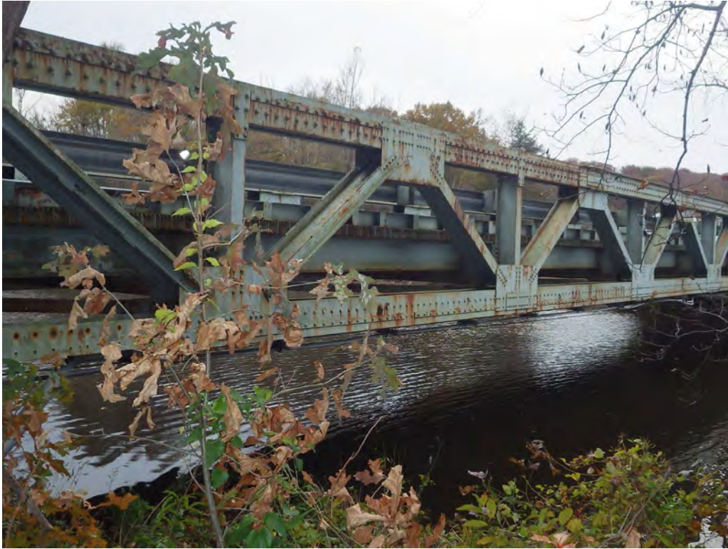
Figure 11. Fracture Critical Element - Typical truss bottom chord and diagonal members (Fracture Critical)
