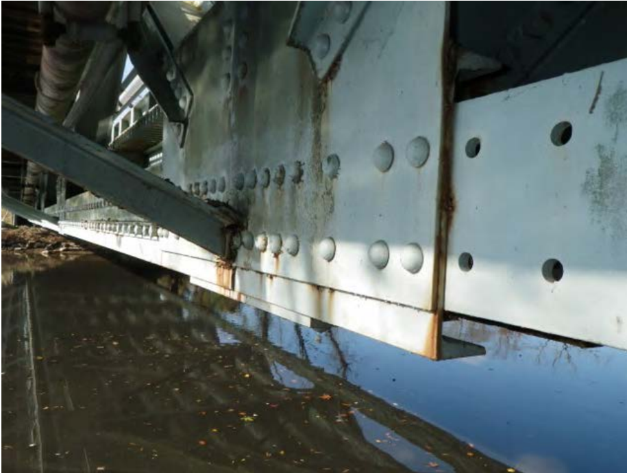
West Sidewalk Handrail Welds to Lower Chord (Fatigue Category C)
