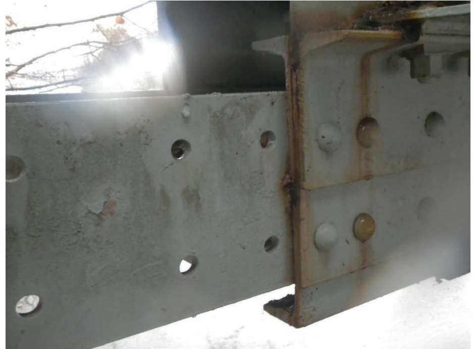
Open holes in lower chord members (Fatigue Category D)
