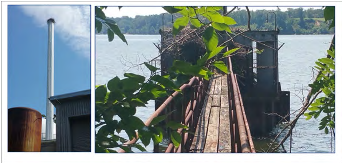
Osprey Nests at the Deactivated SM-1 Nuclear Reactor Facility (USACE, 2019c)
