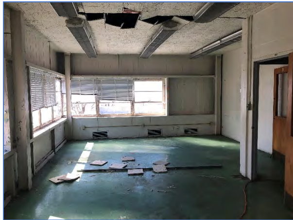
Existing interior space condition in Building 372.
