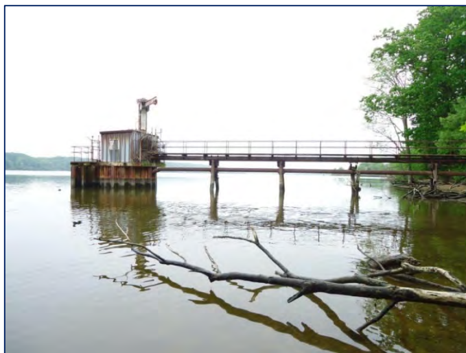
SM-1 Intake Pier and Pump House (USACE, 2019c)
