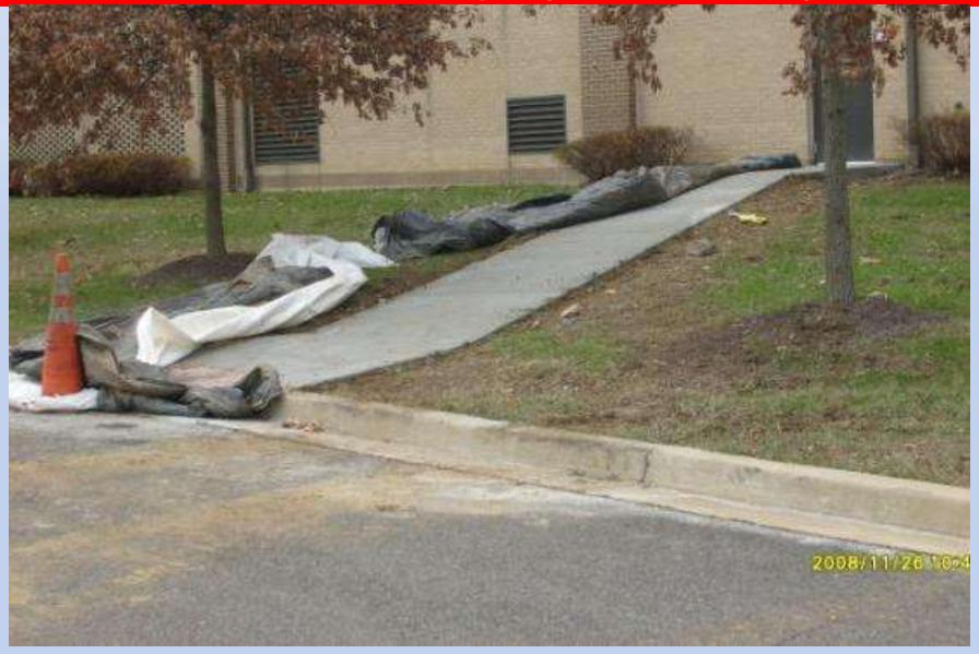
RISE 46 5/8". RUN 36' 10". Jackhammer it and try again. Rise cannot exceed 30" without installing a landing. A rise of 30" must be over 30 feet of ramp length. This situation requires a two-section ramp with midpoint landing. Total length 47 feet plus a 5 foot midpoint landing = 52 feet plus upper landing
