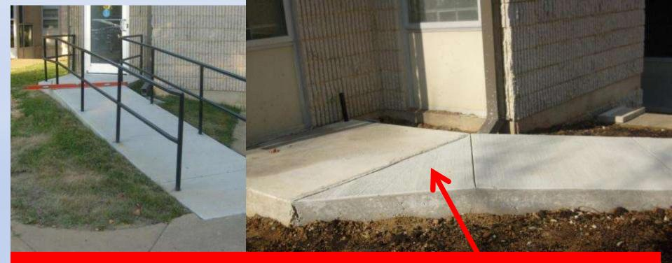
Third try was done correctly. Triangle transition is flat to the landing. Beginning of ramp is 90° to landing.
