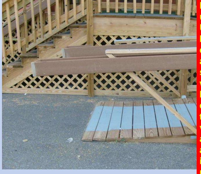
More ugliness. **Using TREX** brand composite as a semi-selfsupporting wooden handrail will cause the rail to fail. Trex is very heavy, and in this application, it is unsupported.
