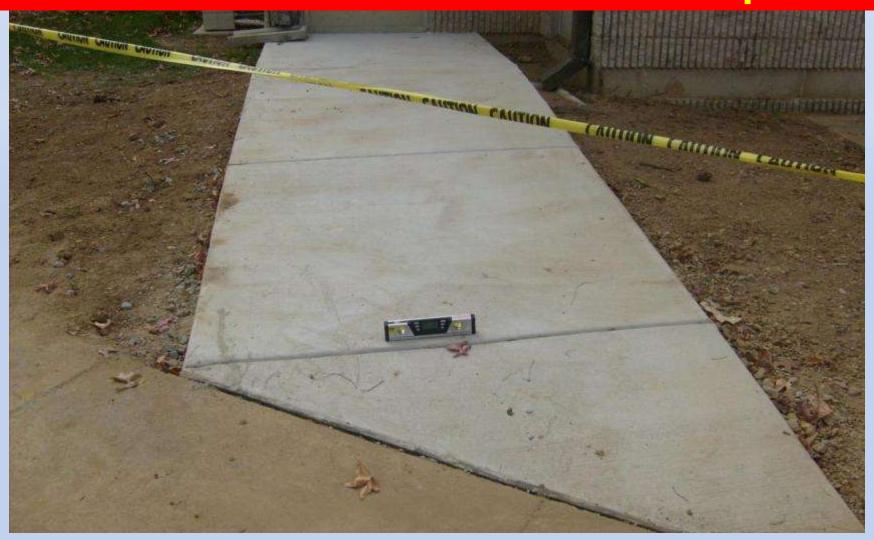
Second attempt. Ramp stretched by angling off to the side. Still missing a 90° transition from the upper landing to the ramp, which caused excessive cross-slope.
