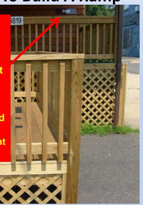
Ramp handrails shall extend past the landing for a distance of at least 12". No sharp, pointy ends allowed!
