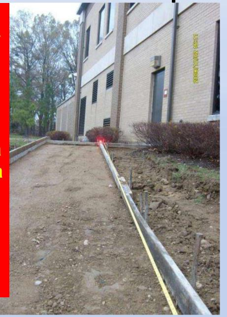
Taped area is a level landing. Failure to make a clean 90° break from the landing to the ramp will result in undesired cross-slope!
