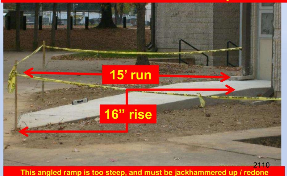
Level shows that the slope of the near-side is different than the slope of the far side.
