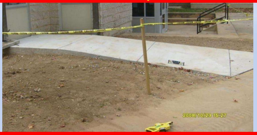
This ramp also has excessive cross-slope
