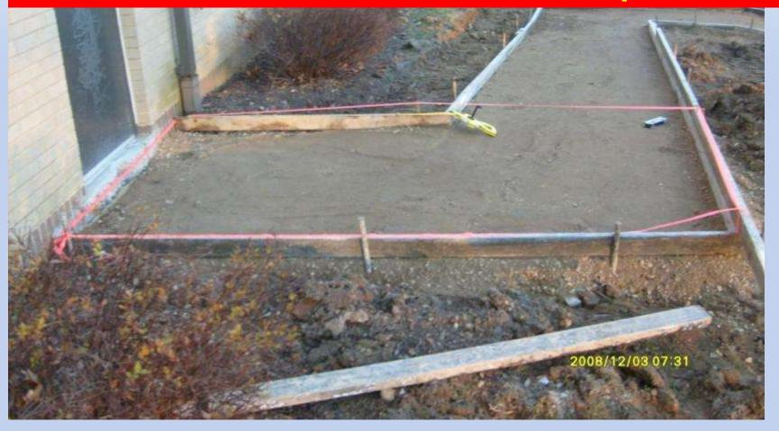
Angled ramp is missing the triangle transition. 6 foot box level is placed where the seam should be, measuring the 2" of elevation change across the ramp. This ramp is illegal, and must be jackhammered up and redone.
