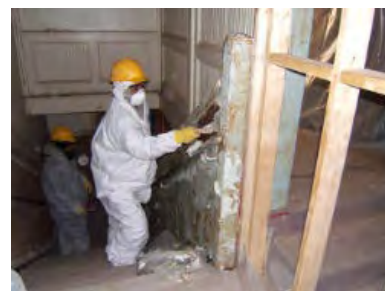
Lead Paint Removal
