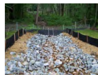
Silt Fence, rip rap, and hay stabilization
