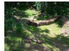
Hay bales and vegetative stabilization
