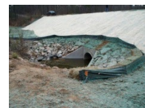
Silt Fence and soil stabilization
