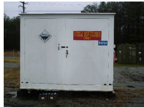
Typical Used Battery Storage Building at DS Maintenance (Bldg 1290)
