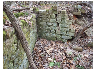
Corner Basement Wall
