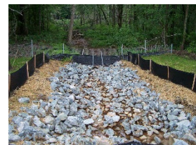
Erosion and Sediment Control
