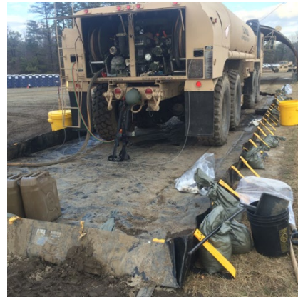
Mobile Secondary Containment
