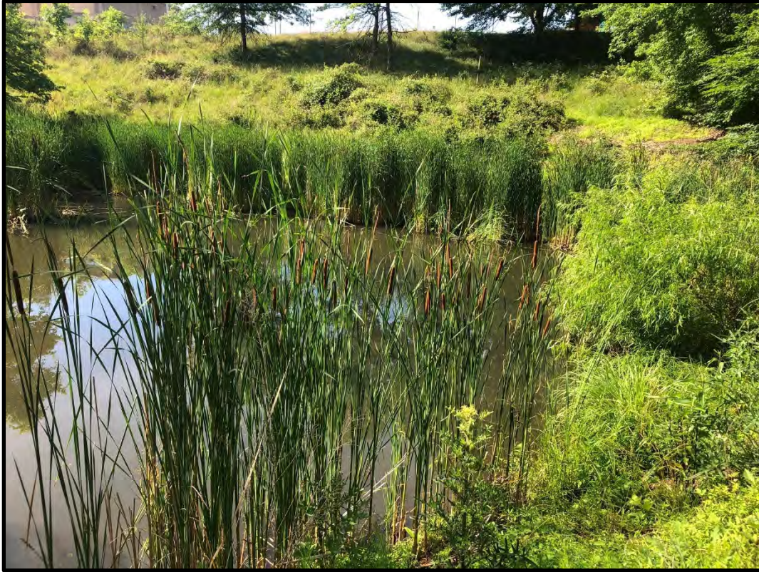
Photo 1: Southwest stormwater pond
