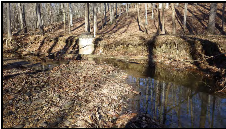
Photo 47: Exposed sewer manhole and erosion on Unnamed tributary, center section
