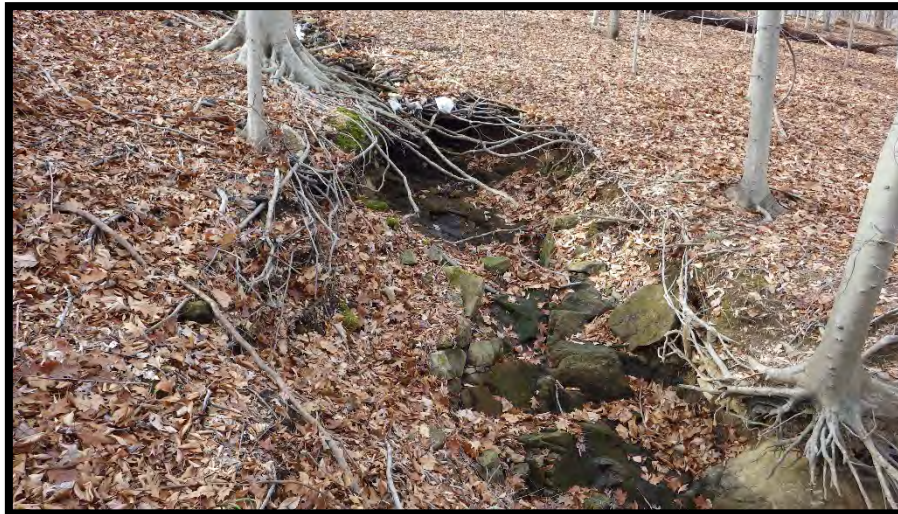
Photo 50: Severe erosion, between outfall and Paint Branch from stormwater outfall in Photo 49
