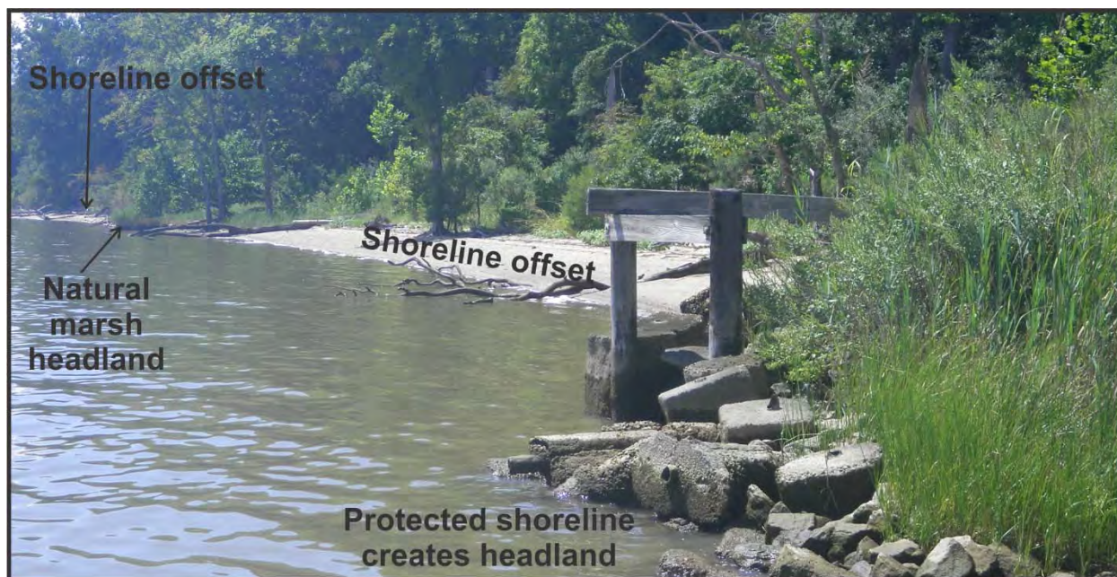
Figure 3-2. Photo of Blossom Point showing how natural and man-made headlands impact the shoreline morphology by creating offsets along the shore. These headlands impact sediment transport along the reach as well.
