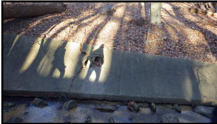
Photo 38: Concrete swale where Hillendale Run flows onto ALC, with two outfalls
