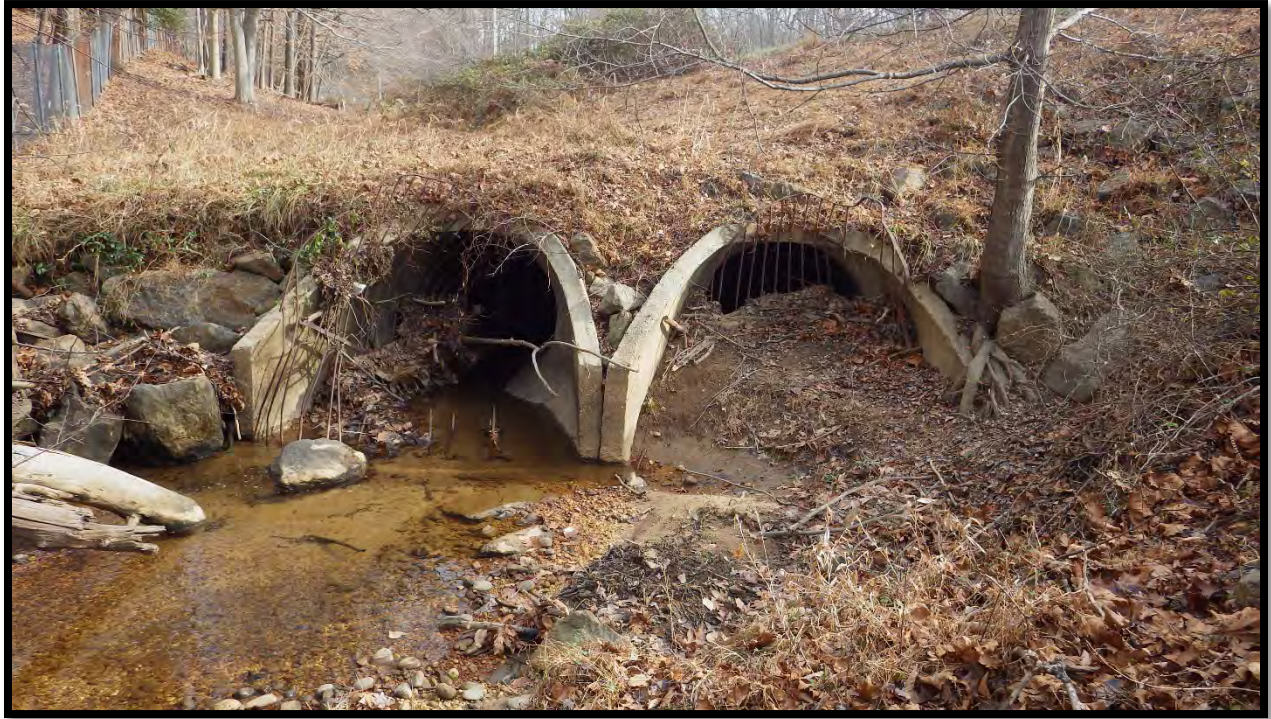
Photo 52: Clogged culverts under Floral Drive on Unnamed tributary, immediately upstream of confluence with Paint Branch
