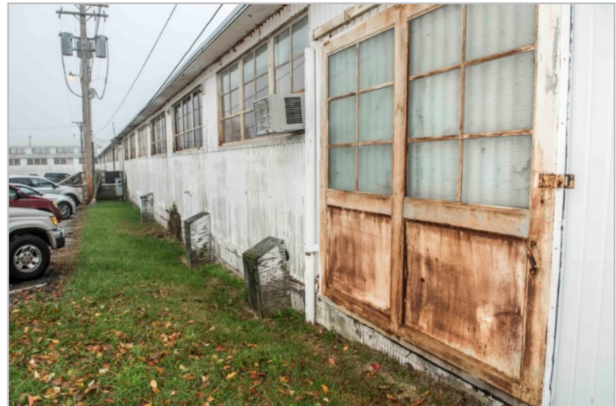
Cement asbestos walls – deteriorating and allow for vermin intrusion and poor HVAC control E-5158
