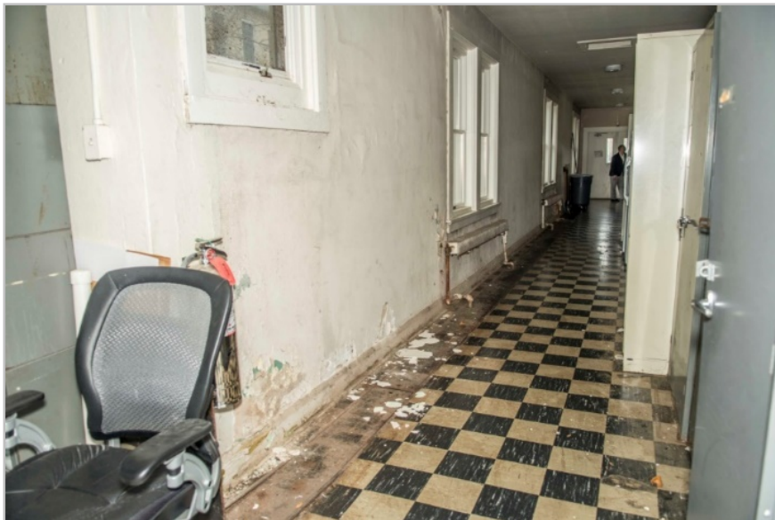
Asbestos tiles and limited storage space (storage cabinets in the hallway) E-1675
