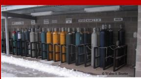
Did you know? Compressed gas cylinders can violently rupture and fail in a fire. Safe storage practices must be adhered to.
