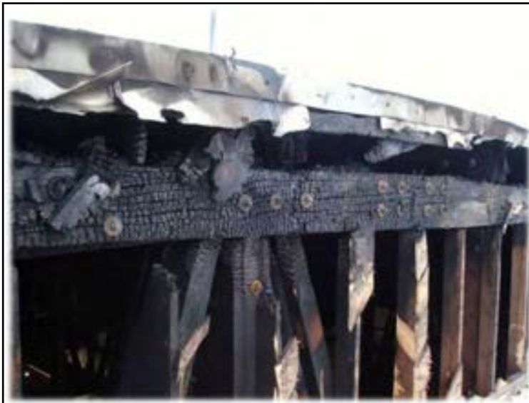
Figure 1-10: Fire Damage Truss #8
