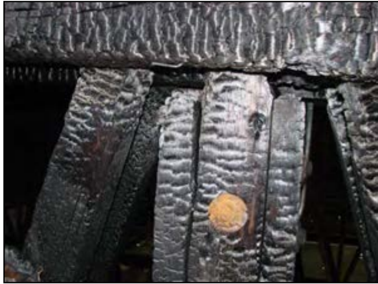
Figure 1-11: Loss of Connectivity Between Members
