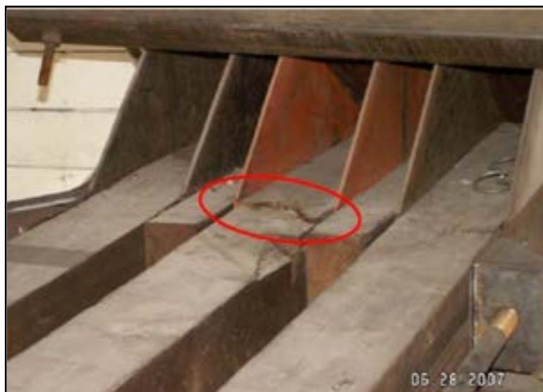
Figure 1-7: Broken Truss Chord – Hangar 3
