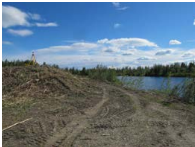
4) Site photo after tree and brush removal showing soil material stockpile and survey-grade GPS control point.
