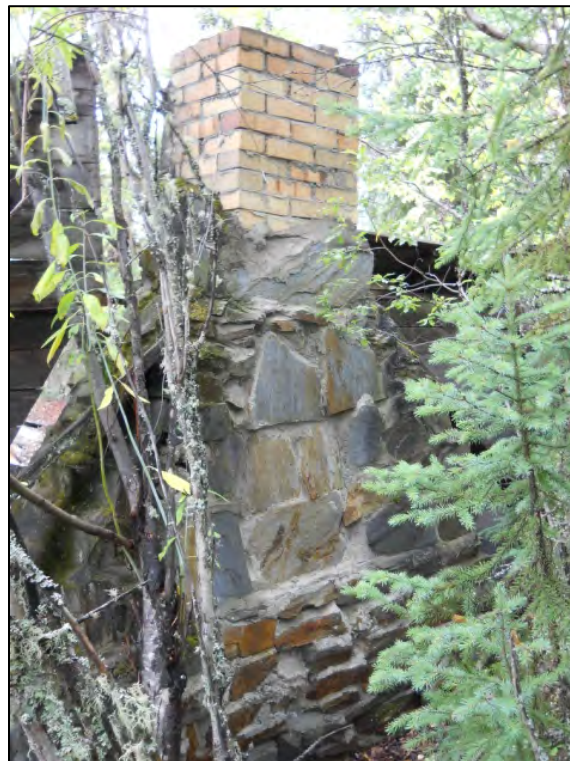
Figure 13. FAI-02198 fireplace with brick layered with mortar and natural rock.
